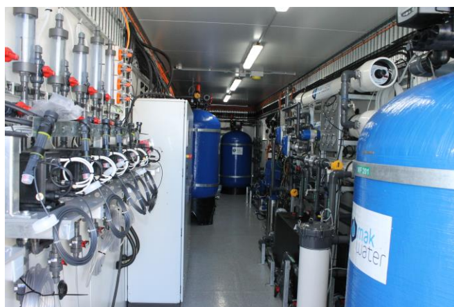
Easily transportable system installed in a sea-container for plug and play onsite installation
