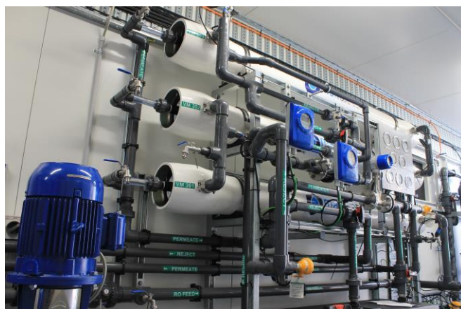
Brackish Water Reverse Osmosis (BWRO) treating contaminated groundwater
